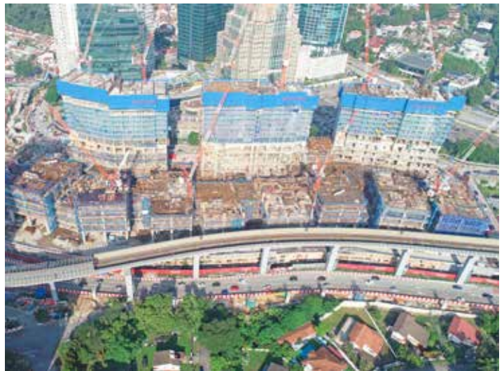
Pavilion Damansara Heights Phase One project site in September 2020
